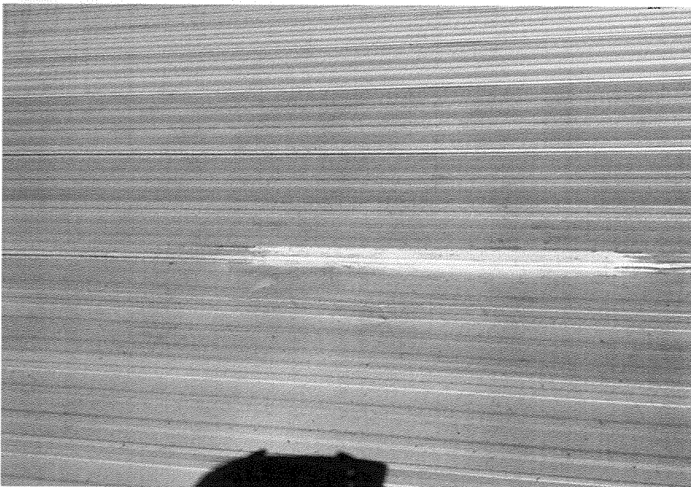
Visible silver coat paint applied over patched areas
