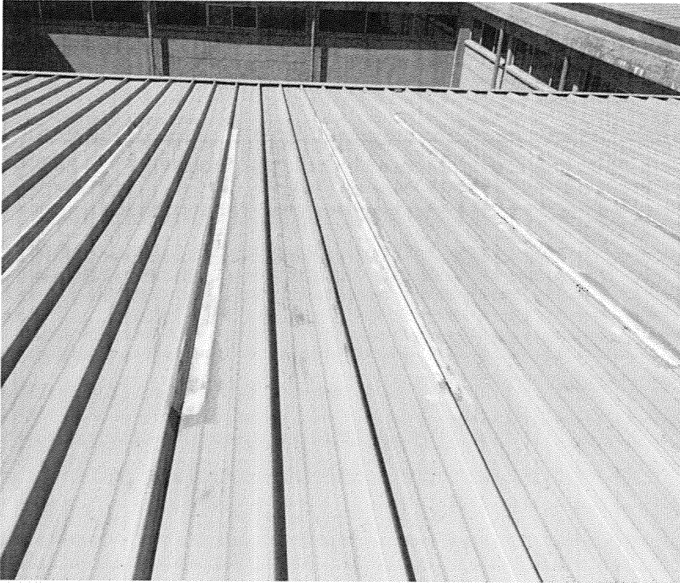
Existing roof patching
