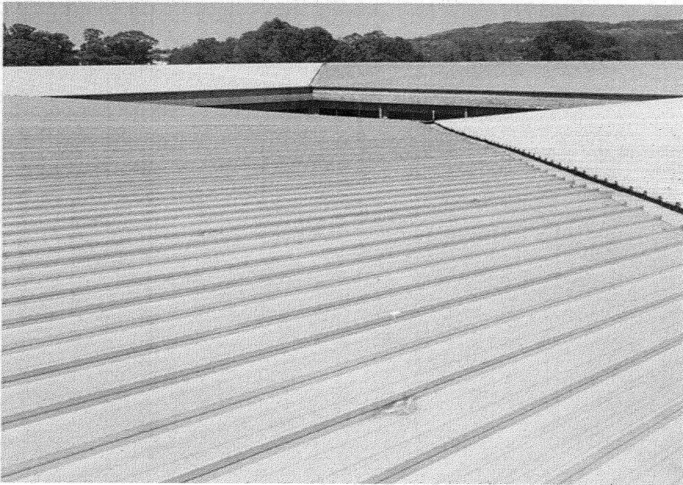
Existing Klip-lok roofing sheet at Enforcement building
